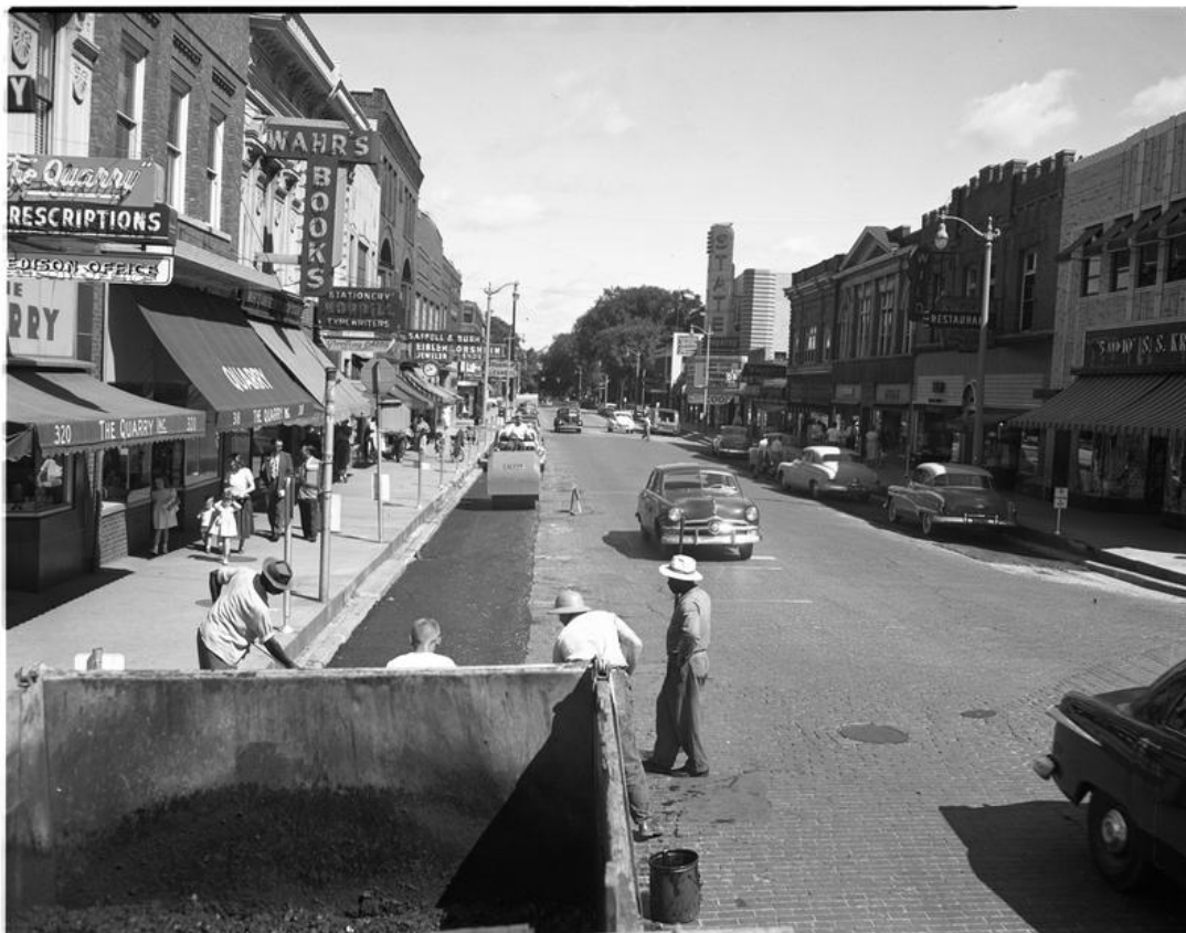
1951 Ann Arbor News photo, paving over the bricks on State Street. Kresge's is on the right.
