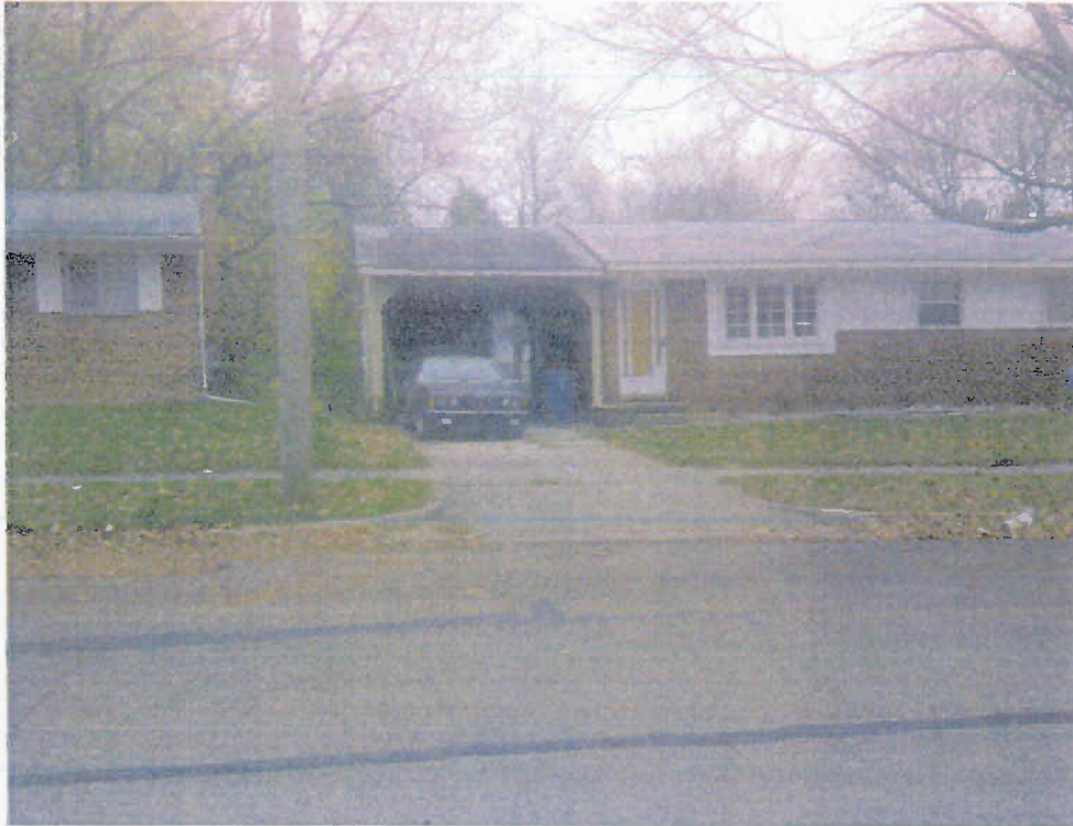
415 Manor – Carport < 5 feet from lot line
