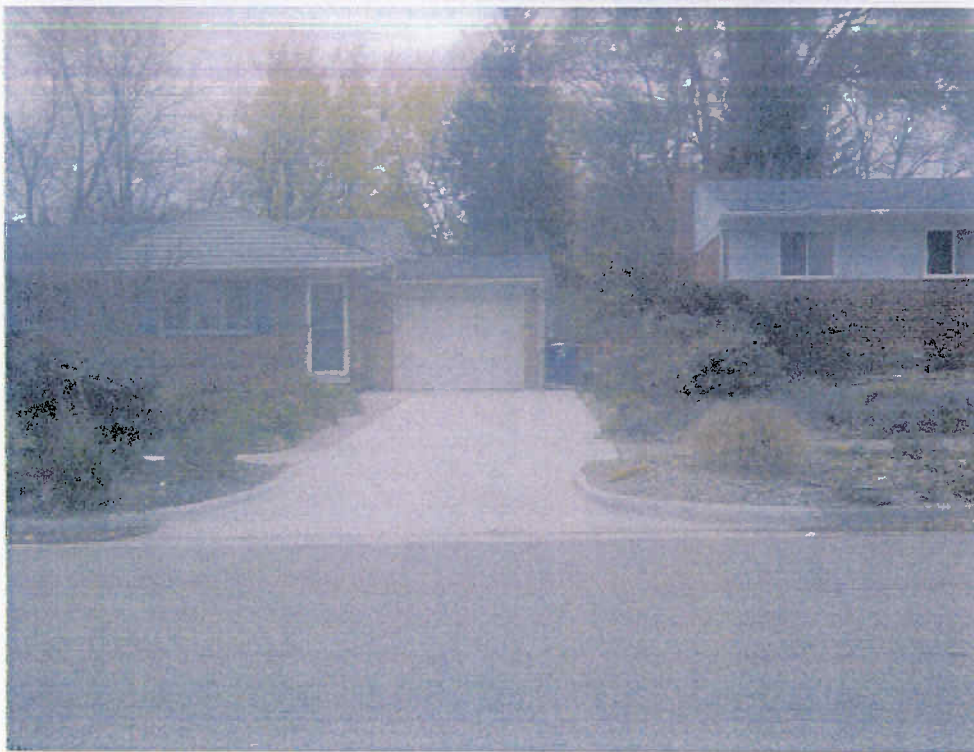
380 Cloverdale – Garage < 5 feet from lot line
