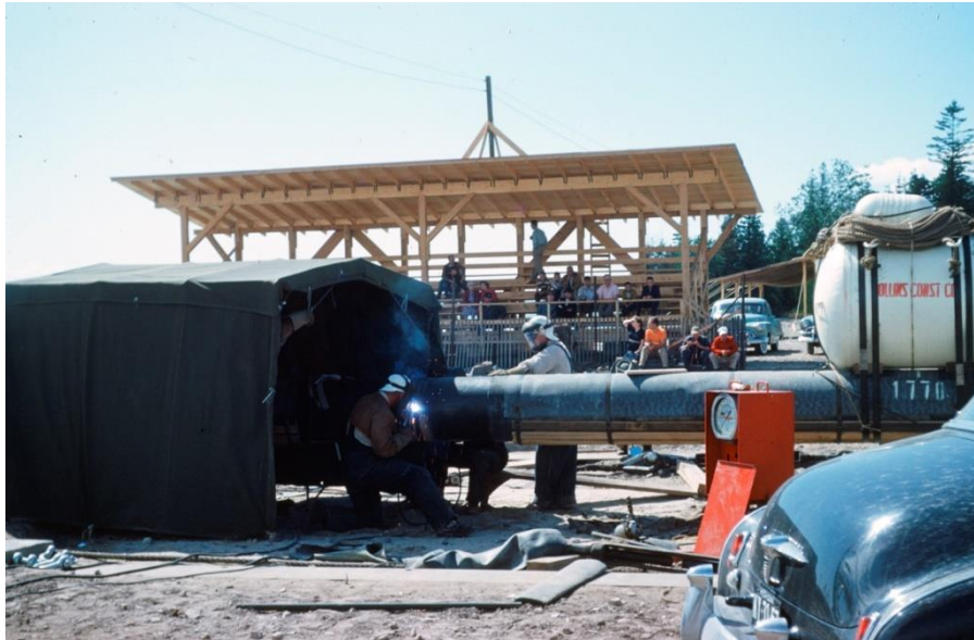
Photo B Trudgen Photo of Pipe String Assembly Welding 0001037005.tif
