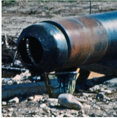
Photo F Detail from Trudgen Photo of Pipe Wrapping Machine 00010370012.tif
