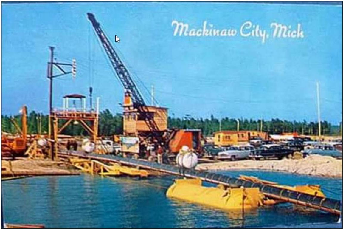
Photo G Postcard of Line 5 Installation Violating Slats Requirement around Entire Pipeline
