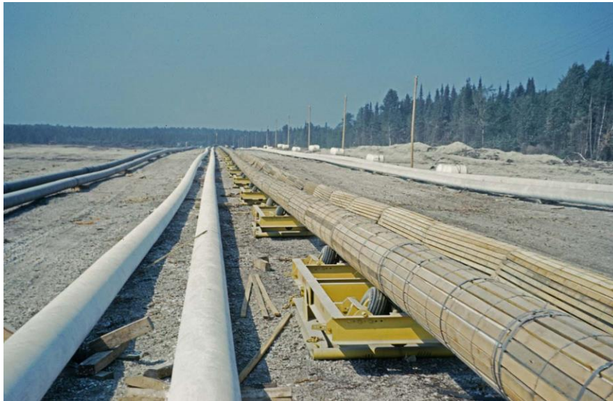
Photo A Trudgen Photo of Pipe Stockyard 00010370011.tif
