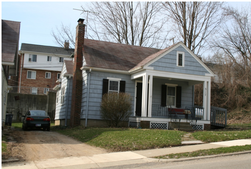
317 Koch Street (April 2008 survey photos)
