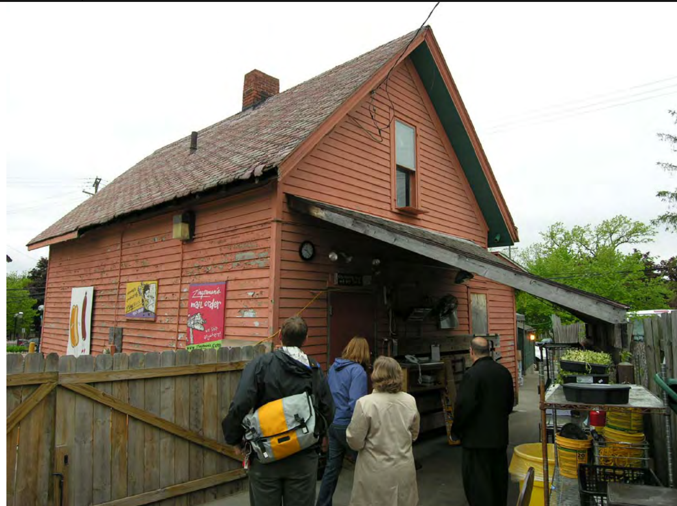
E1 SOUTH EAST CORNER
