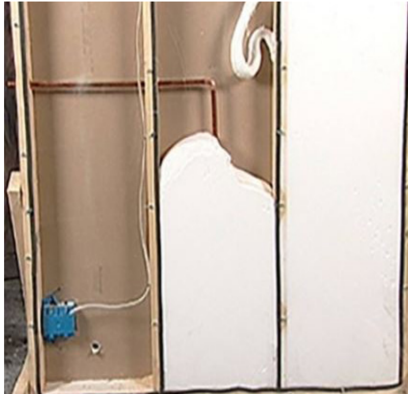
Injection Foam Insulation
