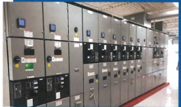
Macomb County, Powerhouse Renovations
