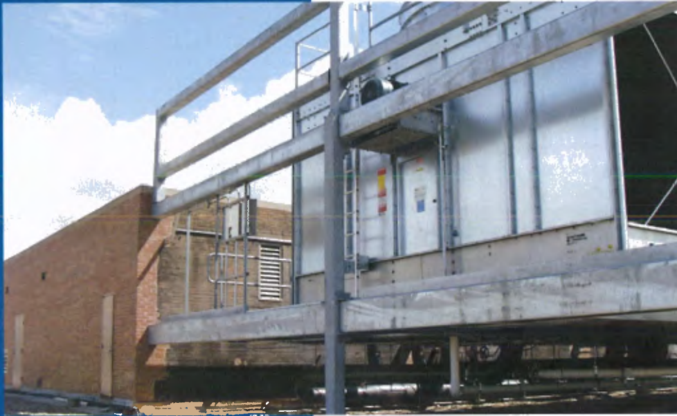
Library Chiller Replacement, Michigan State University
