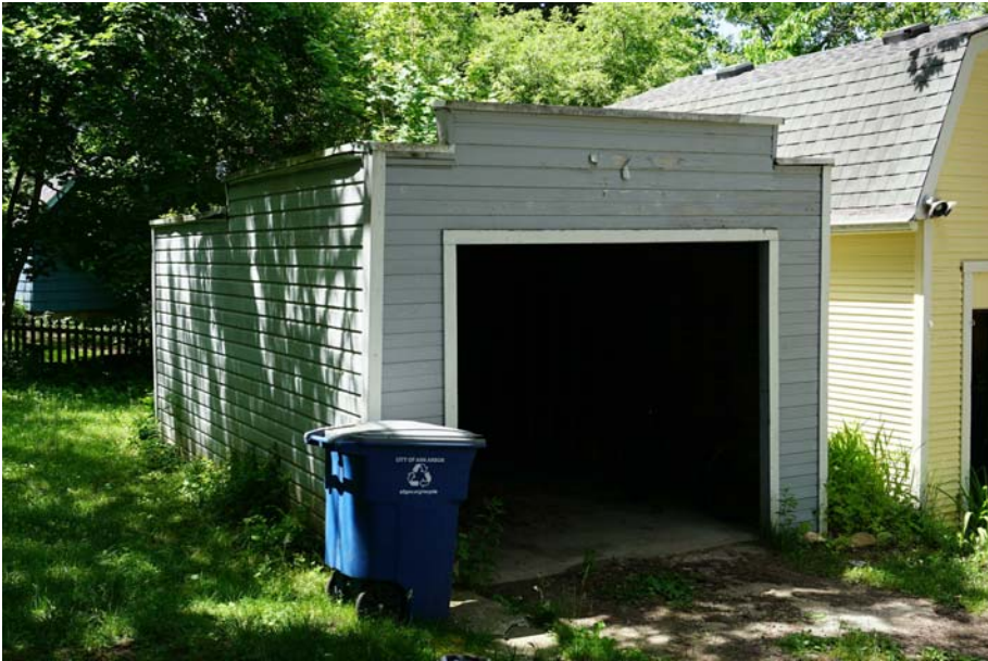
Garage from Southeast
