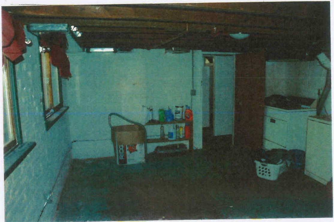
Room #13 exit to hallway to interior stairs
