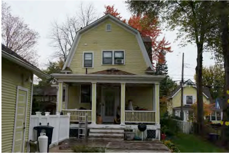
TOP PHOTO OF ORIGINAL 2 STORY HOUSE - EAST SIDE.
