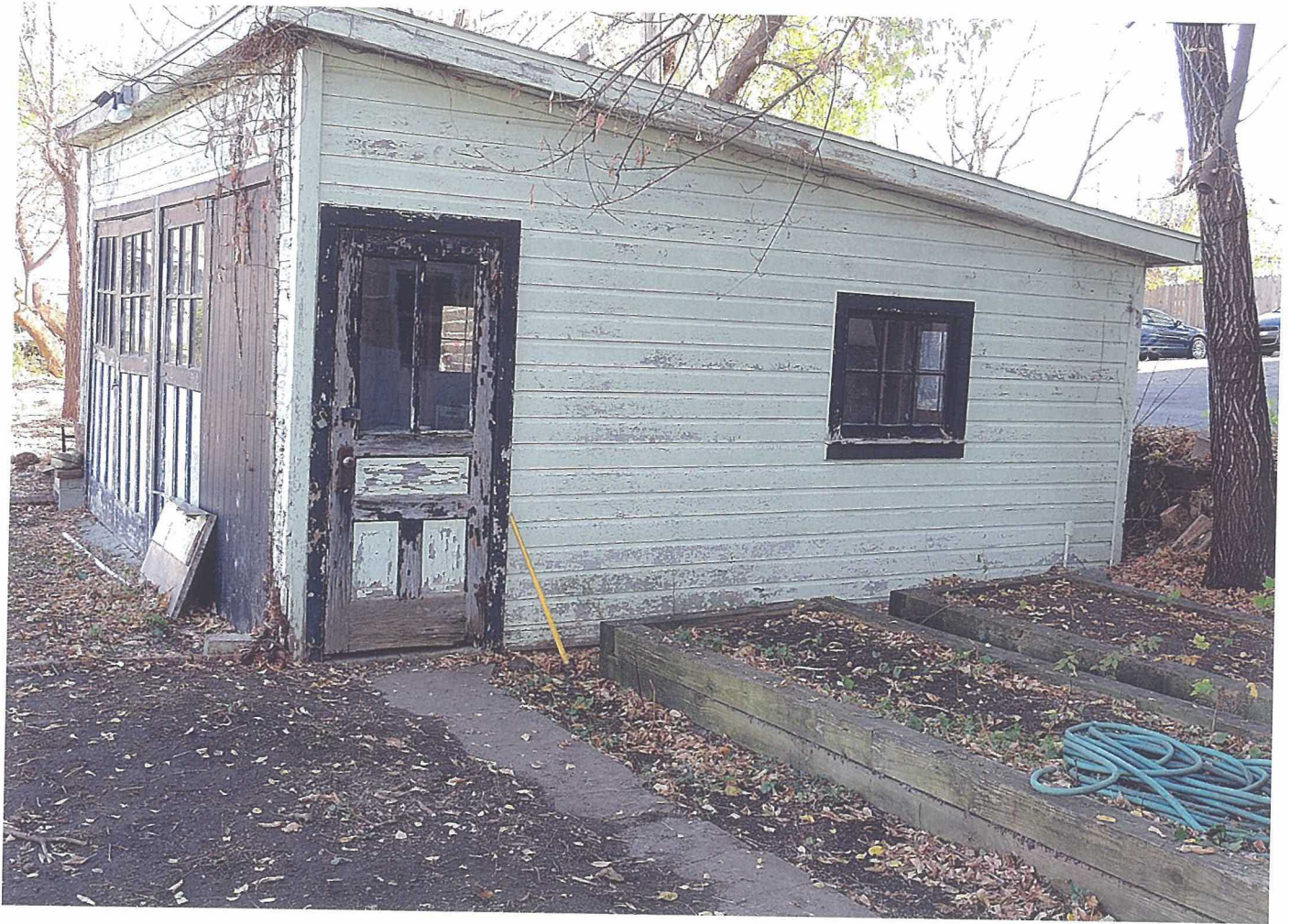
GARAGE (WEST & NORTH)
