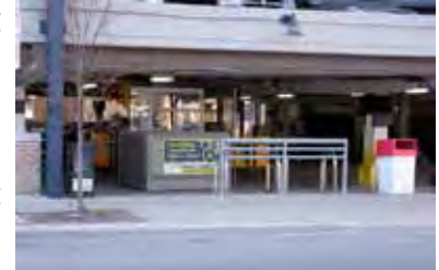
The bottom floor of the 4th & William Parking Structure along Fourth Ave.
