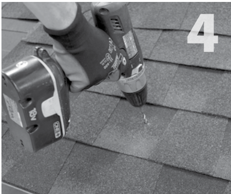
4 Using drill with 7/32" bit, drill pilot hole into roof and rafter, taking care to drill square to the roof. Do not use mount as a drill guide. Drill should be 'long style bit' aka 'aircraft extension bit' to drill a 3" deep hole into rafter.
