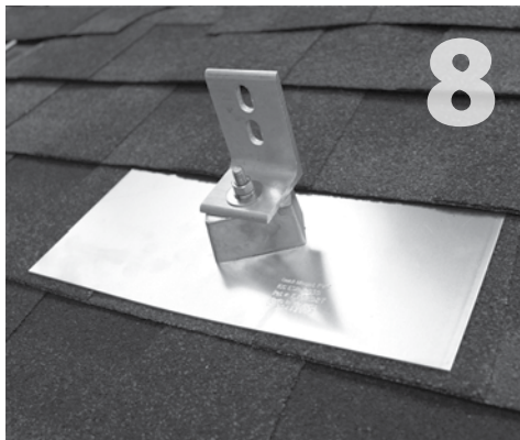
8 Using the rack kit hardware, secure the racking (L-foot) to the mount using torque specs from racking manufacturer. If racking manufacturer does not specify torque setting, tighten to 13 ft.-lbs.
