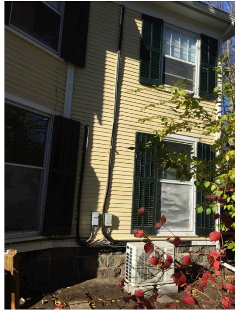
Mini-split compressors and line-sets on the east side of the house.
