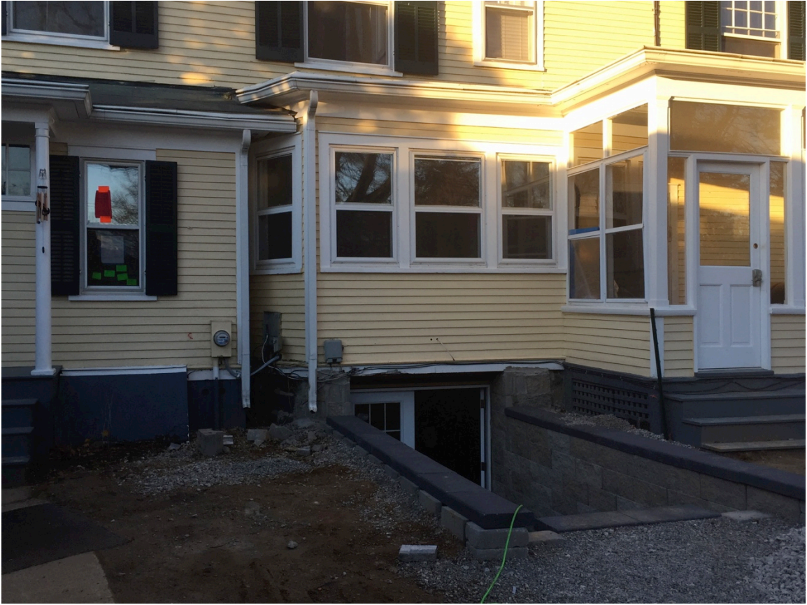
The south entrance to the basement under development.
