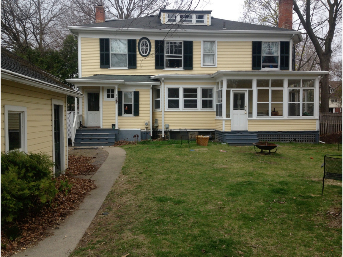
View of the rear of the house prior to the basement construction.
