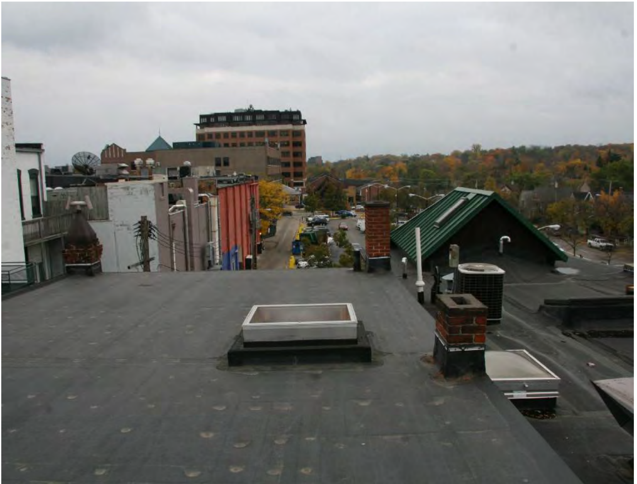
113 W. Liberty Roof, Looking South 12/2013
