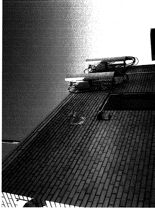
CURRENT SOUTHERLY VIEW
