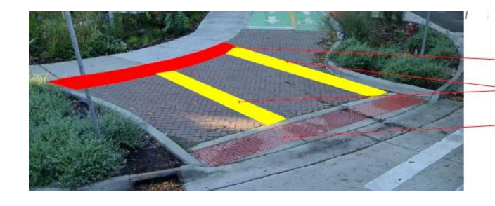
REMOVE 1S FT X 2FT BRICK PAVER FOR TRUNCATED DOMES PER CITY OF ANN ARBOR STANDARD. CLEAN CONCRETE BASE FOR NEW 4" CONCRETE PAVEMENT MATCHING EXISTING ON ALL SIGES. EMBED TRUNCATED DOMES INTO NEW CONCRETE PAVEMENT. 2" WIDE X 15 LONG X 4"THICK.
