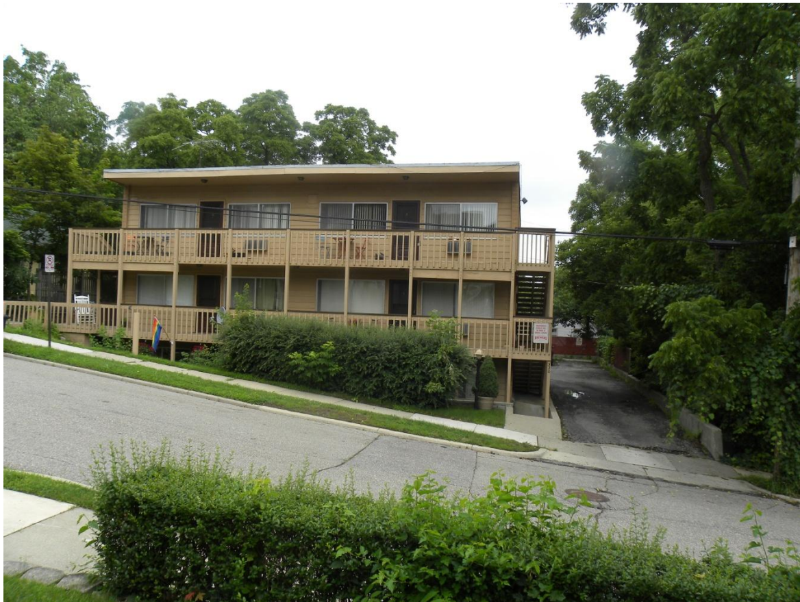
Apartment across Koch (north side)
