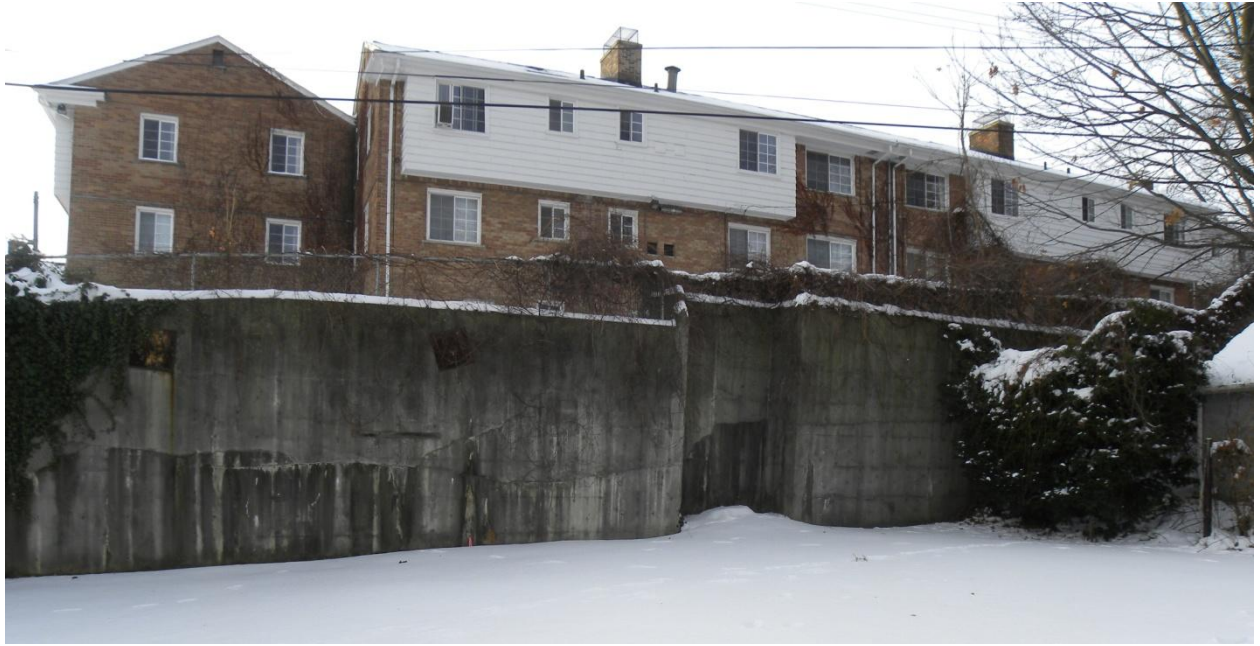
Retaining wall & Knob Hill apartments to the south
