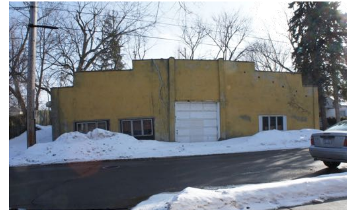
photo above: North Elevation of 211 W. Davis
