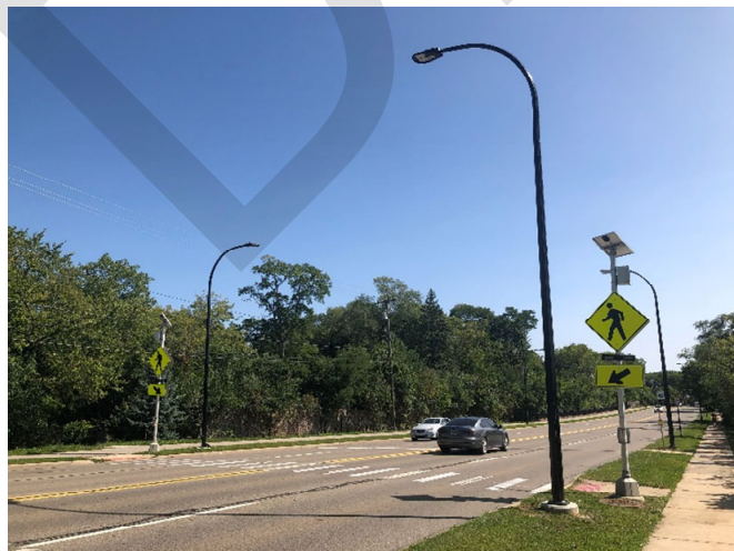
Figure 7 Near Tappan Middle School, crosswalk, with an RRFB, crosses four lanes of traffic with a 45 MPH speed limit with a 30 MPH school zone from 7:30 – 8:20 AM and 3:05 – 3:35 PM
