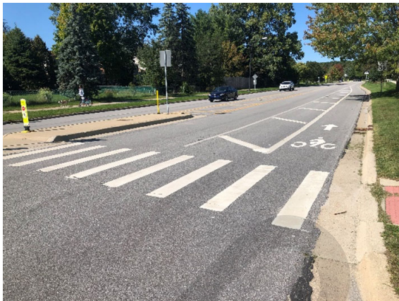
Figure 2 This crosswalk at Green Road and Burbank Road applies high-visibility continental pavement markings.
