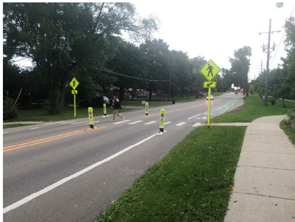
Figure 3 The crosswalk at Pontiac Trail south of Arrowwood Trail has four in-lane pedestrian signs.
