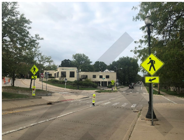
Figure 4 The crosswalk at Broadway and Division includes one in-lane pedestrian sign in the street and one on the island to the left.
