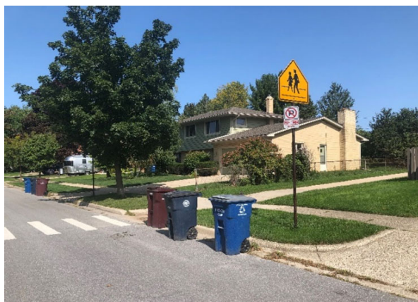
Figure 6 A yellow school warning series sign at Delaware Drive between Mershon Drive and 7th Street. While the yellow color is permitted on MUTCD signage, school warning signs shall have a fluorescent yellow-green background.
