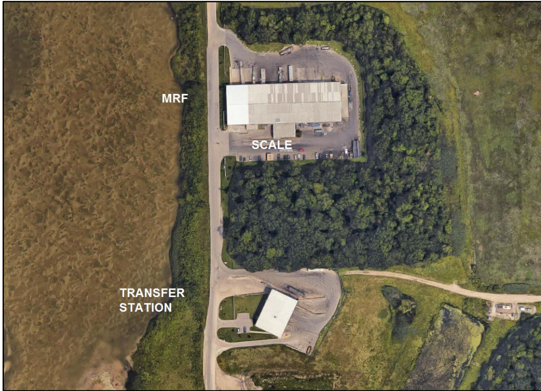
FIGURE 1. AERIAL VIEW OF TRANSFER STATION
