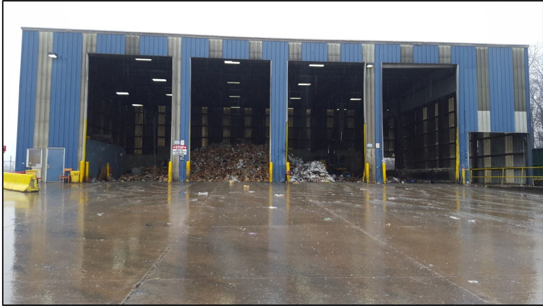
FIGURE 2. VIEW OF TRANSFER STATION BAYS
