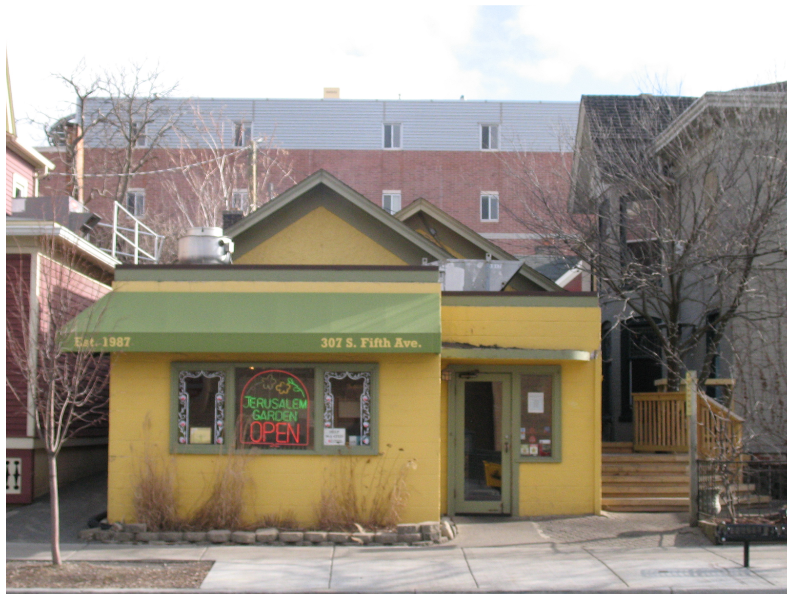
FRONT (WEST) ELEVATION, SHOWING 20 TH CENTURY ADDITION ON EARLIER STRUCTURE, APPARENTLY RESIDENTIAL IN CHARACTER.
