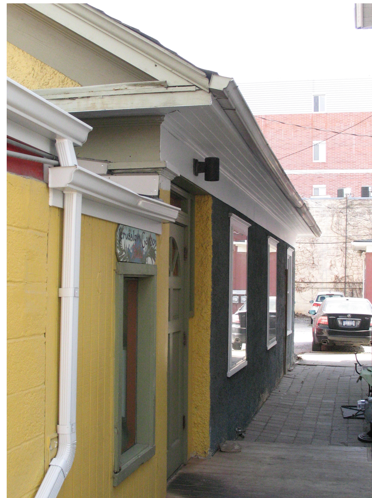
SOUTH ELEVATION FROM WEST.
