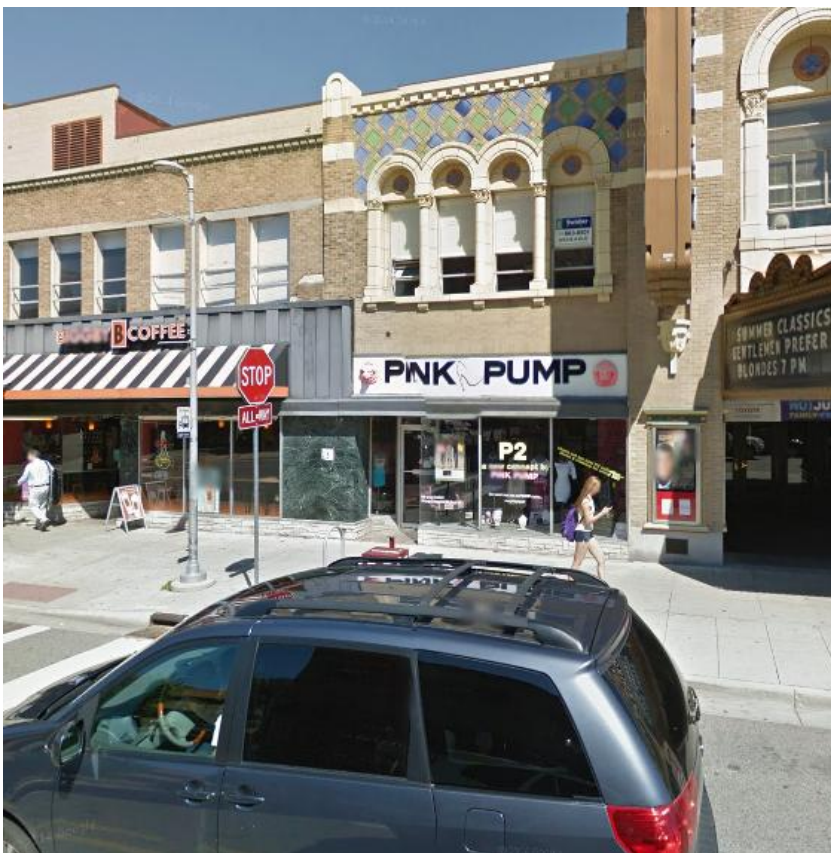
601 East Liberty Street (Google Street View 2012)
